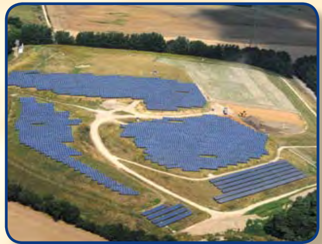
Photovoltaik-Anlage Stralendorf Deponie.
